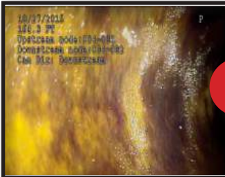
4. Accelerant Burns, Called Out As 'Discolored', But Leaks.
