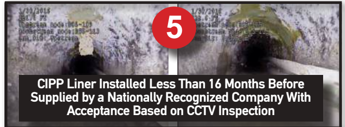
5. Bad Resin. Installed less than 16 months prior.
