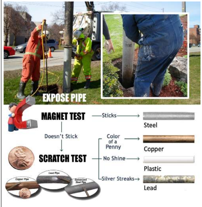
Figure 2. Visual Inspection of Exposed Pipe to Test for Lead Pipe.
