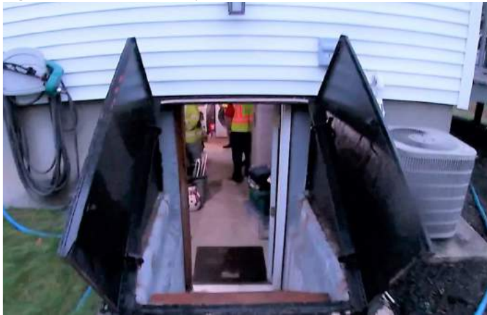
Figure 28. A Basement Entry in Massachusetts.
