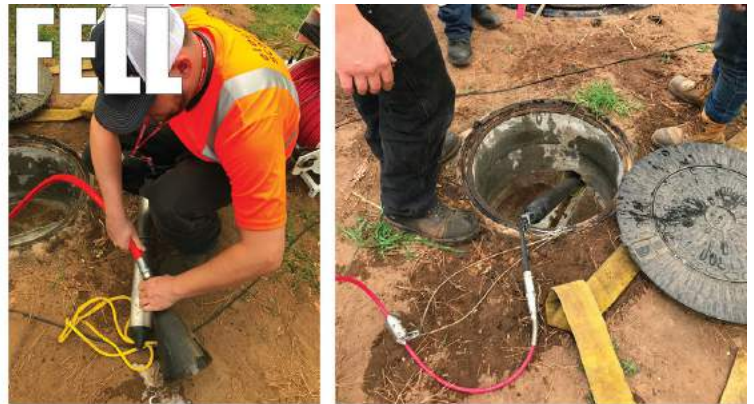
FELL = FOCUSED ELECTRODE LEAK LOCATION
