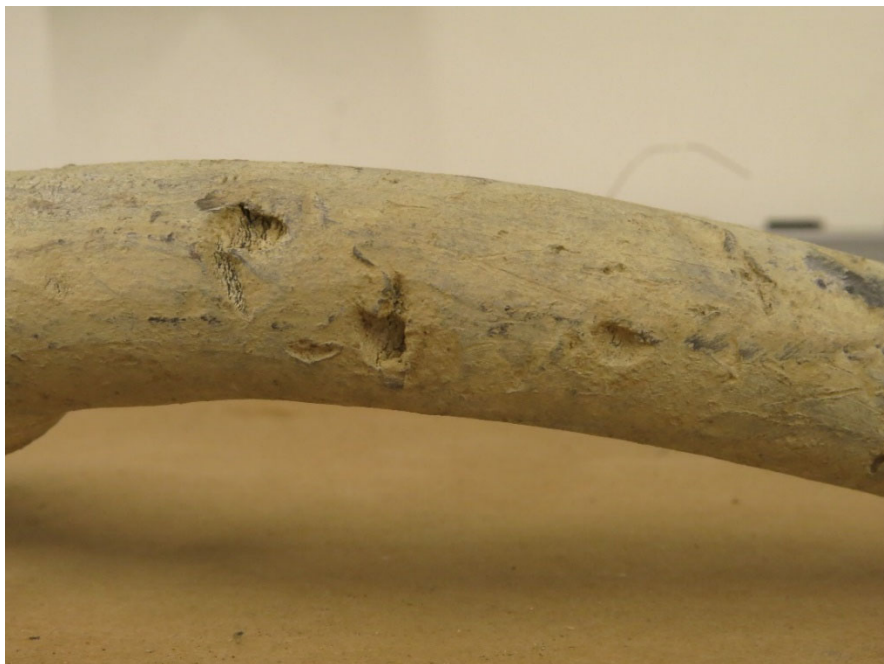
Figure A-15. Damages on the Surface of the Lead Pipe from Sample 16-0209-CP-1.
