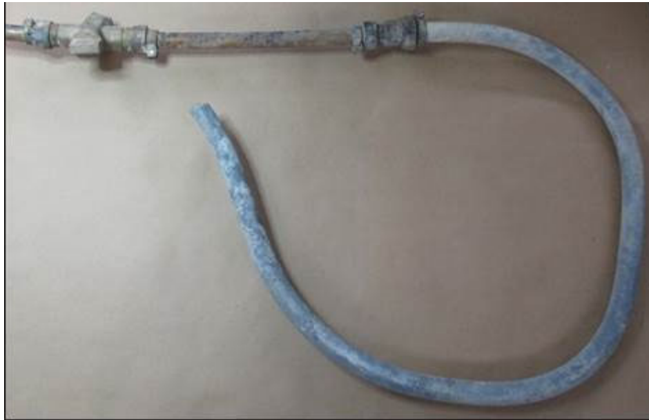
Figure A-8. Sample 16-0209-CP-4, Copper and Lead Pipe with Curb Stop Valve.
